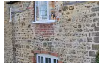
Exposed rubble with red brick dressing
