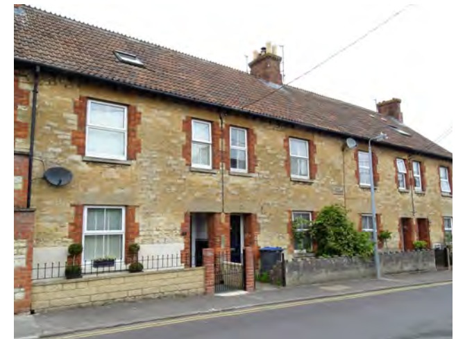
Figure 30: Terrace houses on Shelburne Road with bathstone facade and red brick decorative features.
