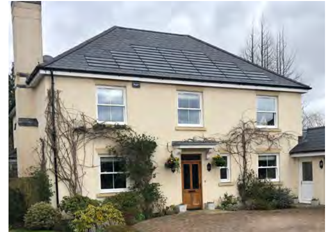
Figure 172: Use of shingle-like solar panels on a slate roof, with the design and colour of the solar panels matching those of the adjacent slate tiles.
