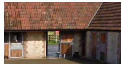
Gabled roof with red clay tiles and yellow stone and red brick
