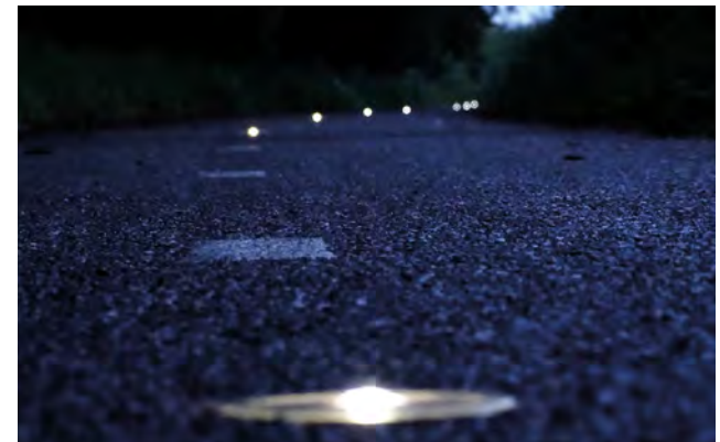
Figure 109: Example of a foot/cycle path which is lit by solar cat's-eye providing some light for pedestrian and cyclists without creating any disturbance to the nearby properties or unacceptable levels of light pollution.
