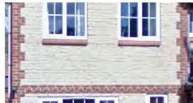
Limestone rubble with red brick dressing
