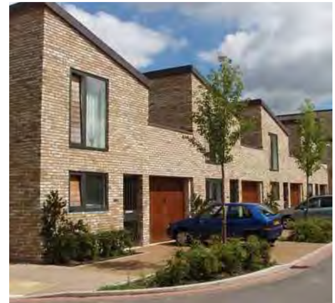
Figure 112: Positive example of on-plot garage parking with vegetation, street trees and permeable paving, Cambridge.
