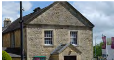
Exposed rubble stone
