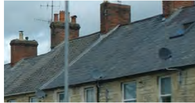
Gabled roof with grey slate tiles
