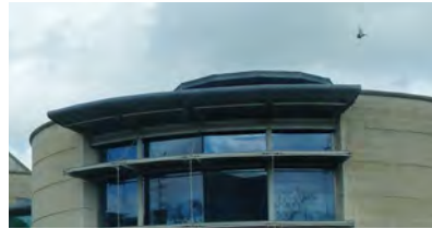
Flat roof with limestone ashlar on façade
