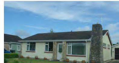
White rendered façade with stone side chimney and local stone bordered doorway
