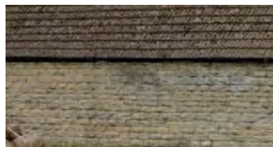
Local stone on façade
