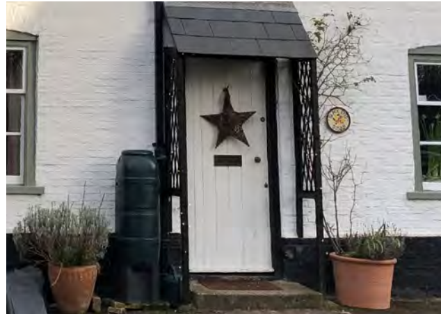
Figure 137: Examples of water butts used for rainwater harvesting in Reach, Cambridgeshire.
