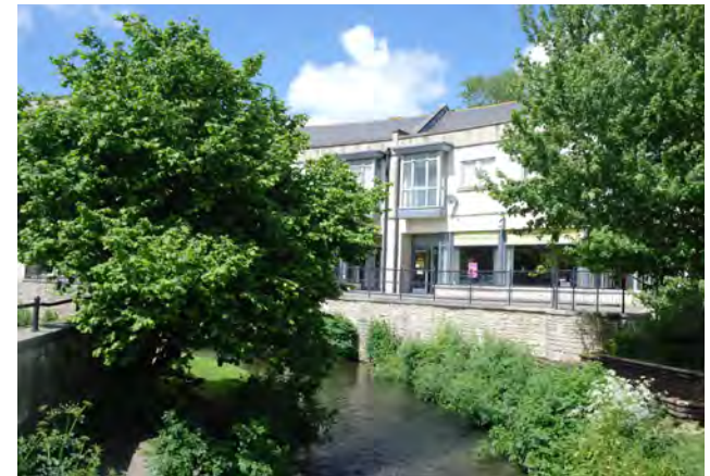
Figure 19: Beach Terrace - a mixed-use development fronting onto the river and Church Street, built during the 1990s redevelopment of Calne Town.
