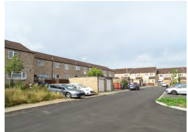
Figure 35: Houses laid out in clusters around the cul-de-sac of Woodroffe Square within the Coleman's Farm estate - another commonly recurring layout across this character area.
