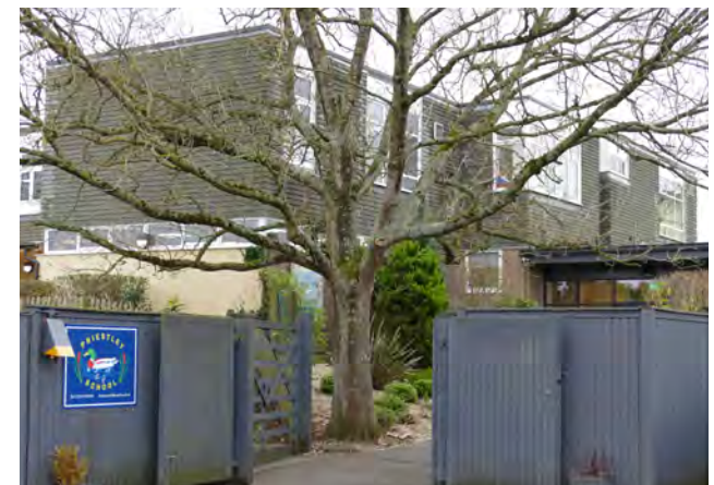
Figure 33: View of Priestley Primary School.
