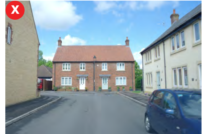
Figure 43: Hardscape-dominated streetscapes with little vegetation and boundary treatments between properties and roads should be avoided in future developments.
