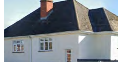
Hipped roof with red brick chimney and white render on façade
