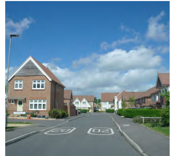
Figure 42: The most recent developments are dominated by hardscaping, some incorporate soft boundary treatment elements to soften the impact - such as grass verges, hedgerows and small trees
