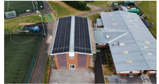
Beversbrook Sports Centre solar panels
