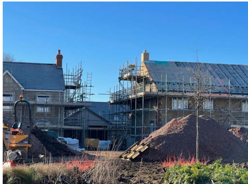
Houses under construction on Stoke Meadow
