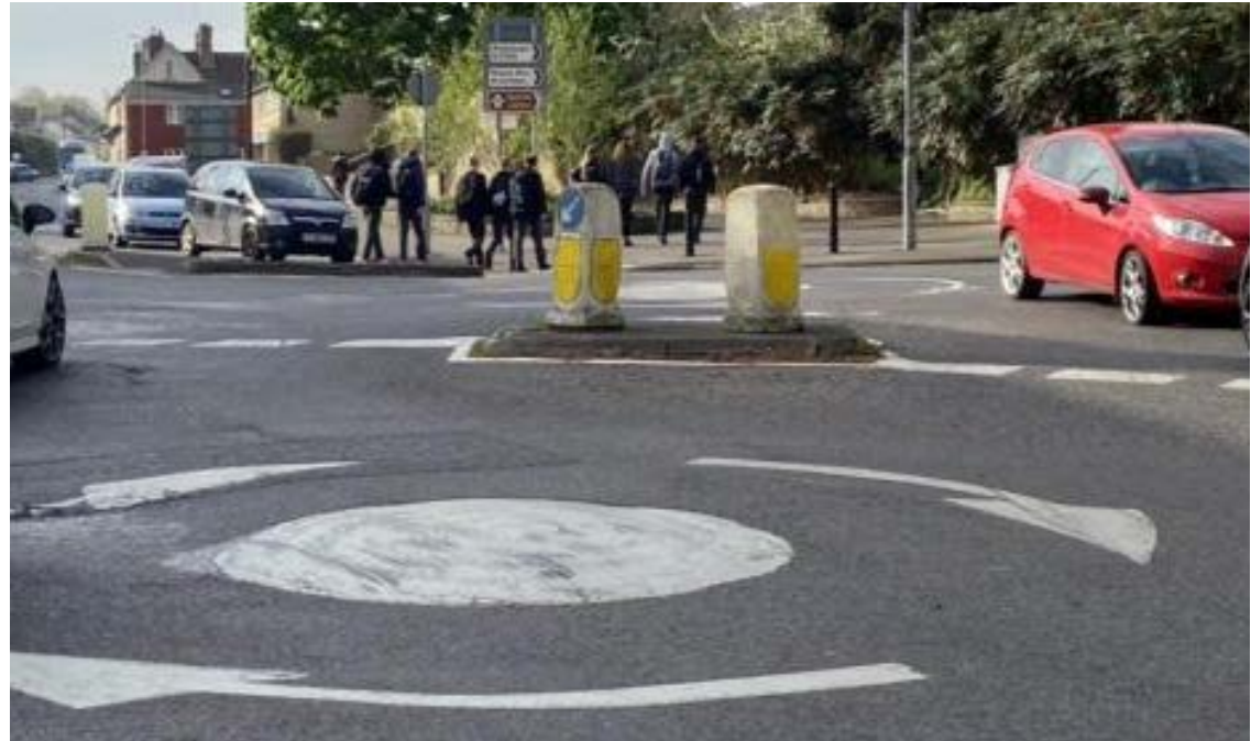
Lack of Pedestrian Crossing at Junction of A4 and Silver Street
